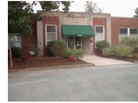
Fork Union School The restrooms are still set up for the little children. It is air conditioned and completely renovated since it was last used as a grammar school.
